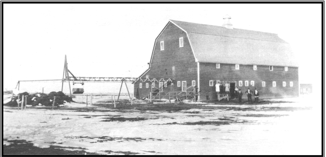
An example of a large dairy barn in the 1930s - This one was equipped with a manure carrier Source: Horndean Reunion Committee, Horndean Heritage , 1984, p.57
